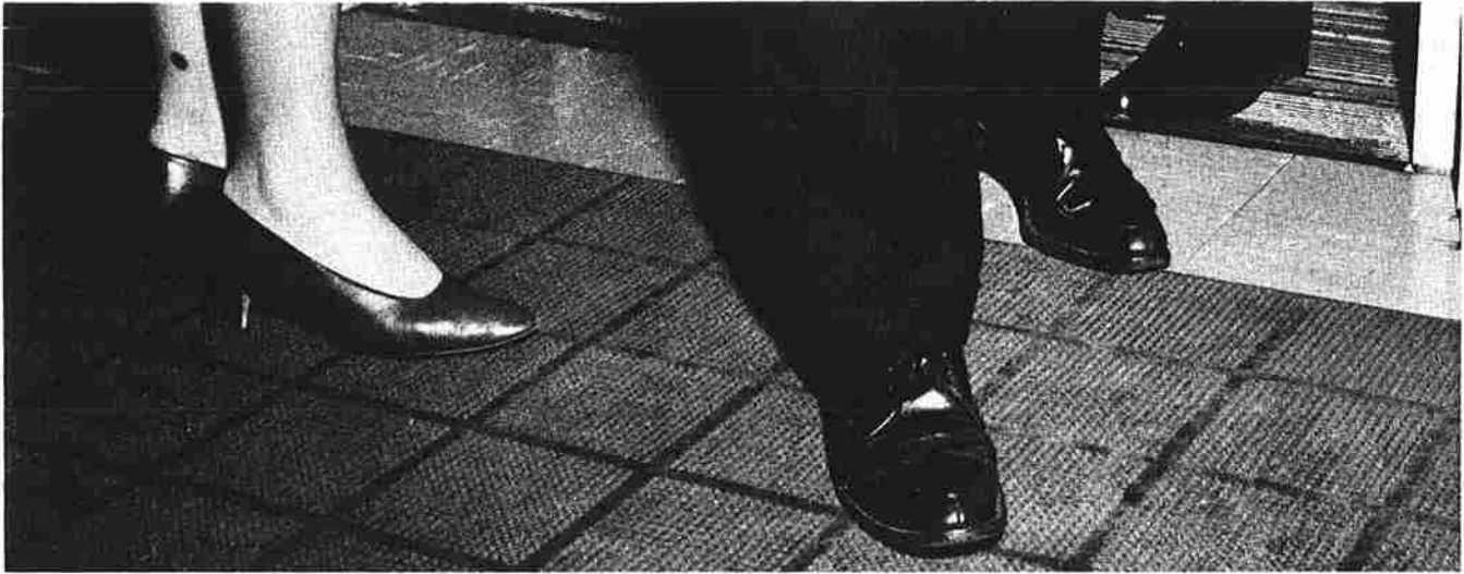
Figure 25-2. A heavyweight rubber or plastic mat with a nubby finish or raised design and beveled edges tends to lie flat and stay in place. Rotating the mat distributes the wear and minimizes 'bald' spots in high-traffic locations.
